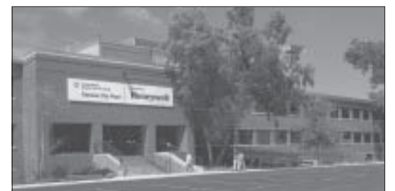
The Kansas City Plant, one of the most unique and diverse manufacturing facilities in the world, is home to leading-edge educational technology.
